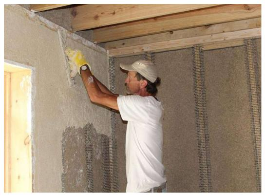
Fig 5.20 Plaster mixture being smooth with a metal trowel
