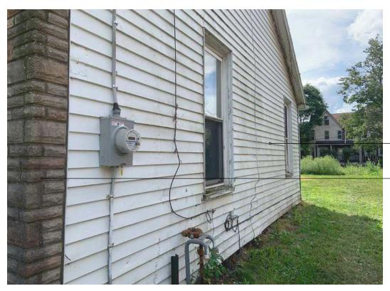
Fig 4.1 Existing exterior with vinyl siding
