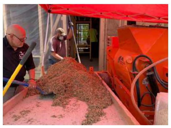
$\textbf{Fig 5.9} \ \textbf{The team then shovels the mixture from the Mud Hog, into the sprayer}$
