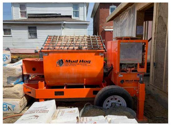
$\textbf{Fig 5.7} \ \text{The install starts with the Mud Hog, which mixes the hemp hurd, lime and water} \\$
