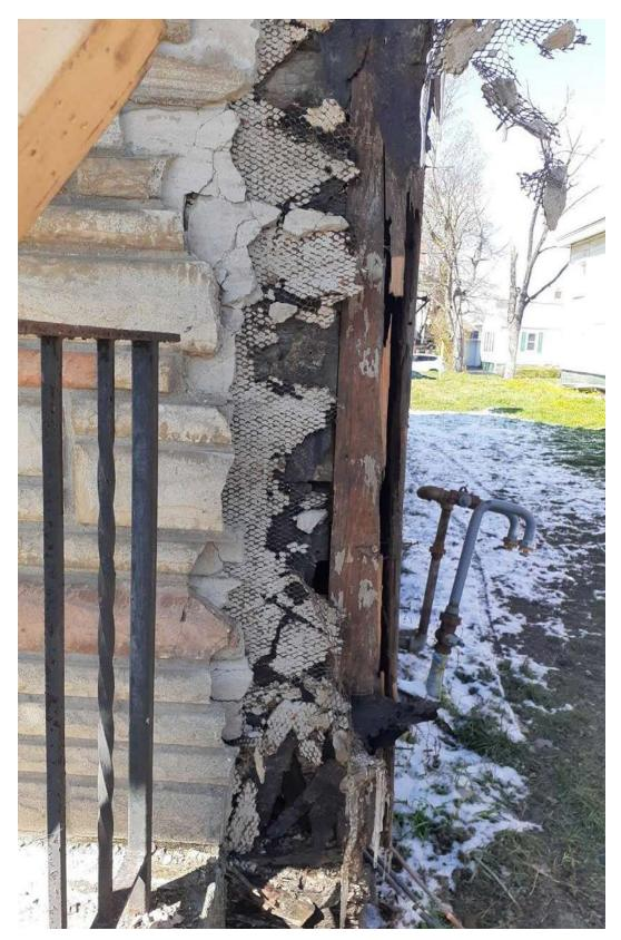
Fig 4.9 Damaged wood and structure at the foundation
