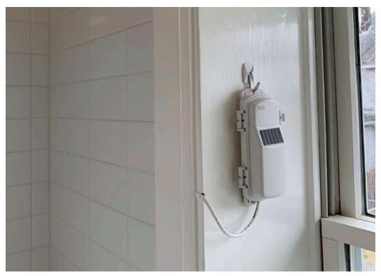
Fig 8.4 Heat flux monitor in the upstairs bathroom that was installed by PHRC
