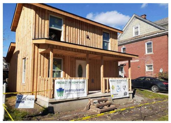
Fig 5.17 PA Hemp Home's exterior with newly installed, locally sourced, hemlock rainscreen
