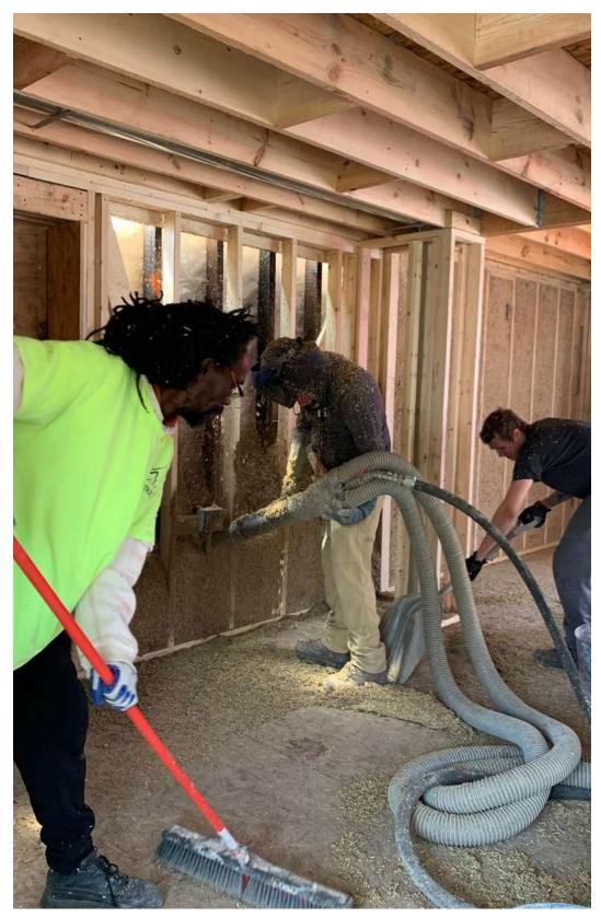
Fig 5.13 On the inside, as the mixture is being installed, a team of two sweeps up the excess and shovels it into a buckets
