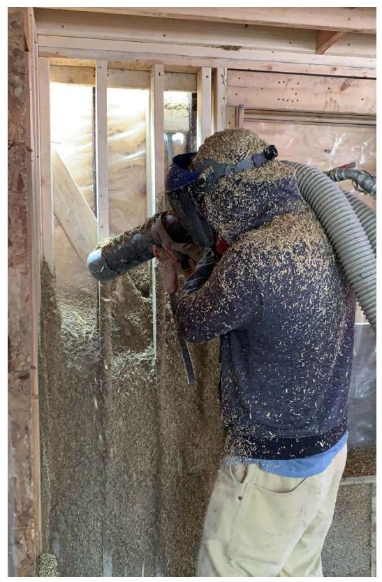
Fig 5.11 Cameron from Americhanvre installing the hemplime mixture
