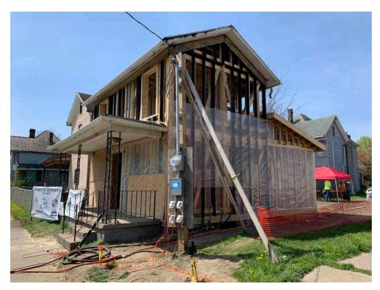
Fig 5.6 The home fully framed and prepped for the spray-applied hemplime install
