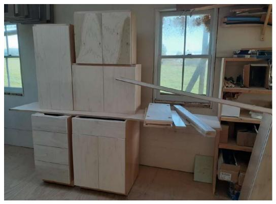
Fig 6.4 Wall and Base Cabinets ready and waiting to be finished with healthier paint
