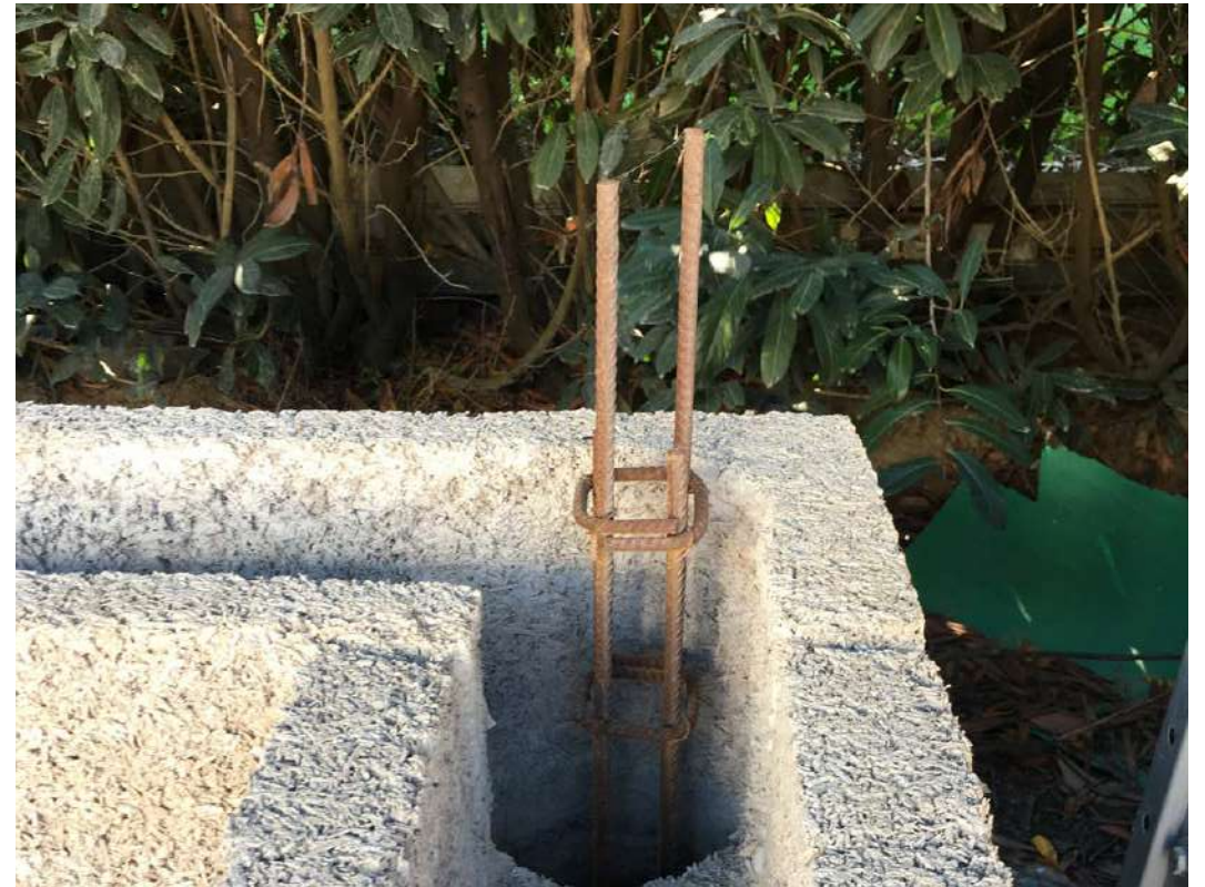
Fig 6.7 Isohemp hemp+lime walls and concrete structure
