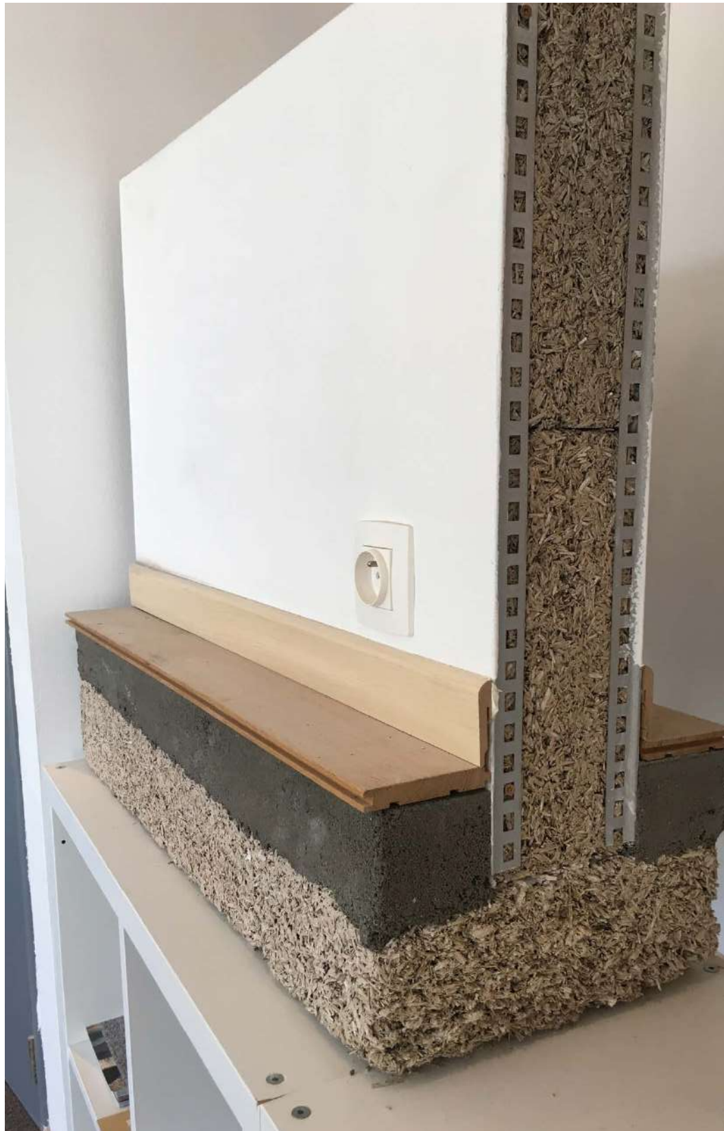
Fig 6.6 Typical hemp+lime interior wall section
