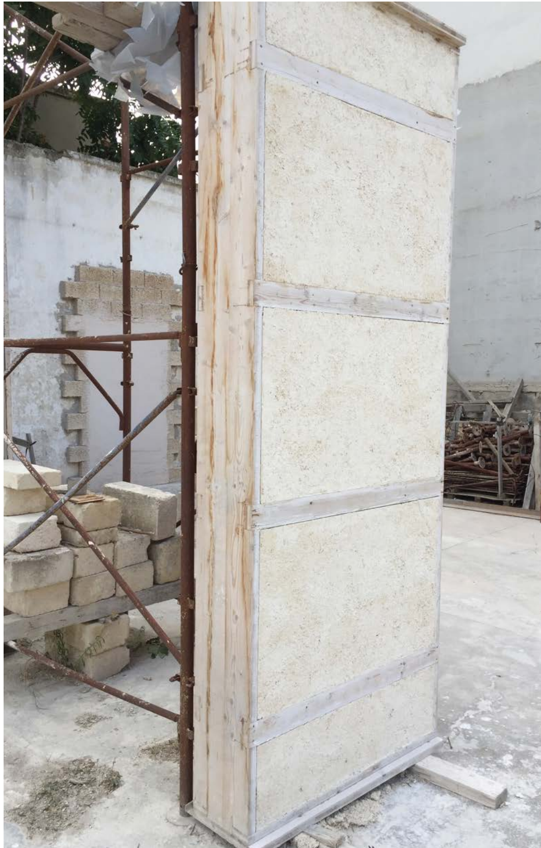
Fig 6.13 Prefabricated hemp+lime wall panels, Puglia, Italy
