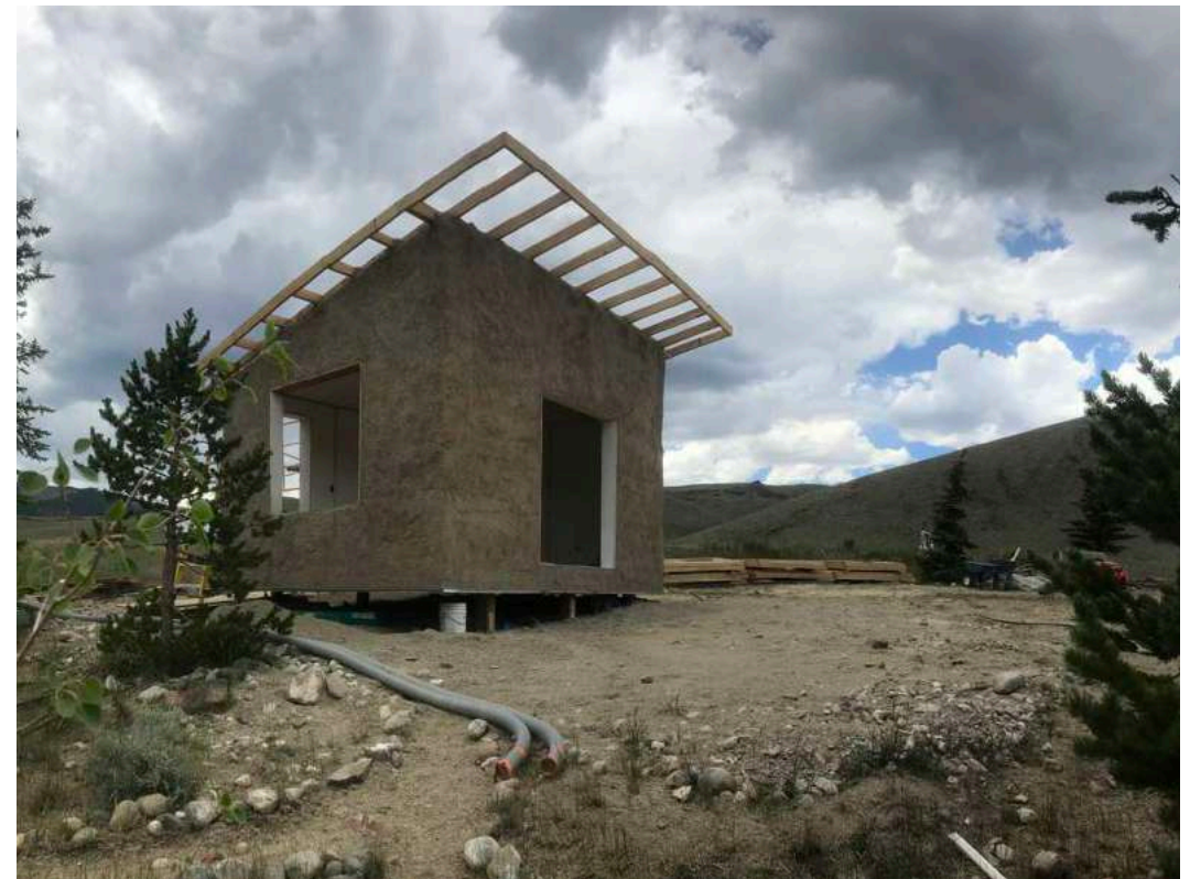
Fig 7.1 Structure using blown hemp+lime
