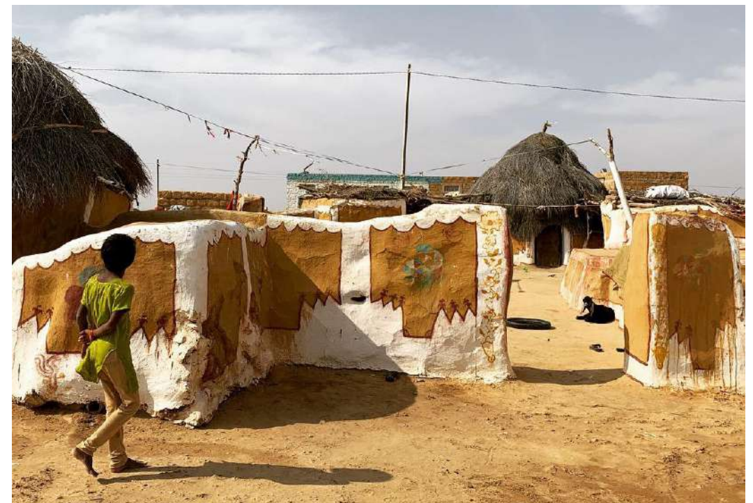
Fig 4.4 Lime paint over cow dung plaster in desert village homes, Jaisalmer, India
