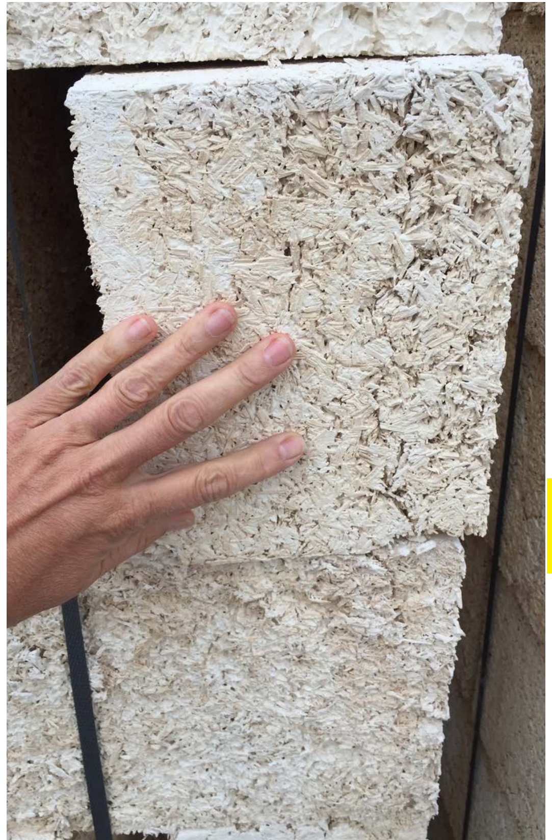
Fig 6.11 Hemp and lime blocks + mortar, Puglia, Italy
