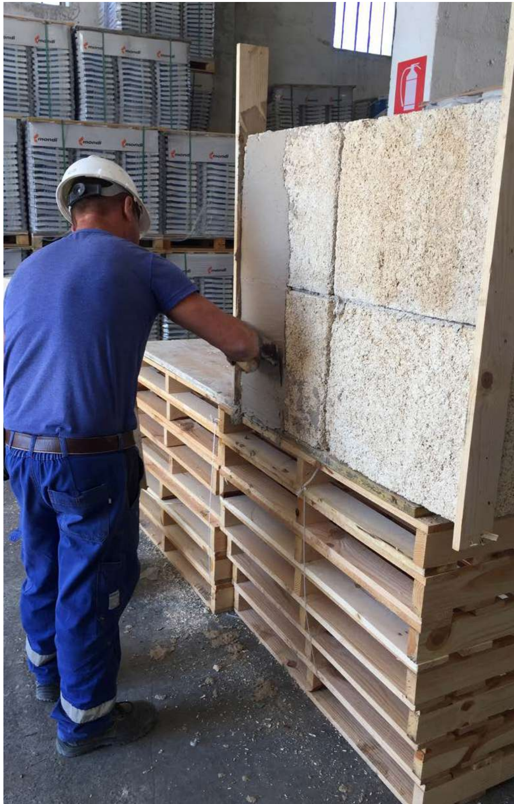
Fig 6.17 Application of hemp and lime blocks
