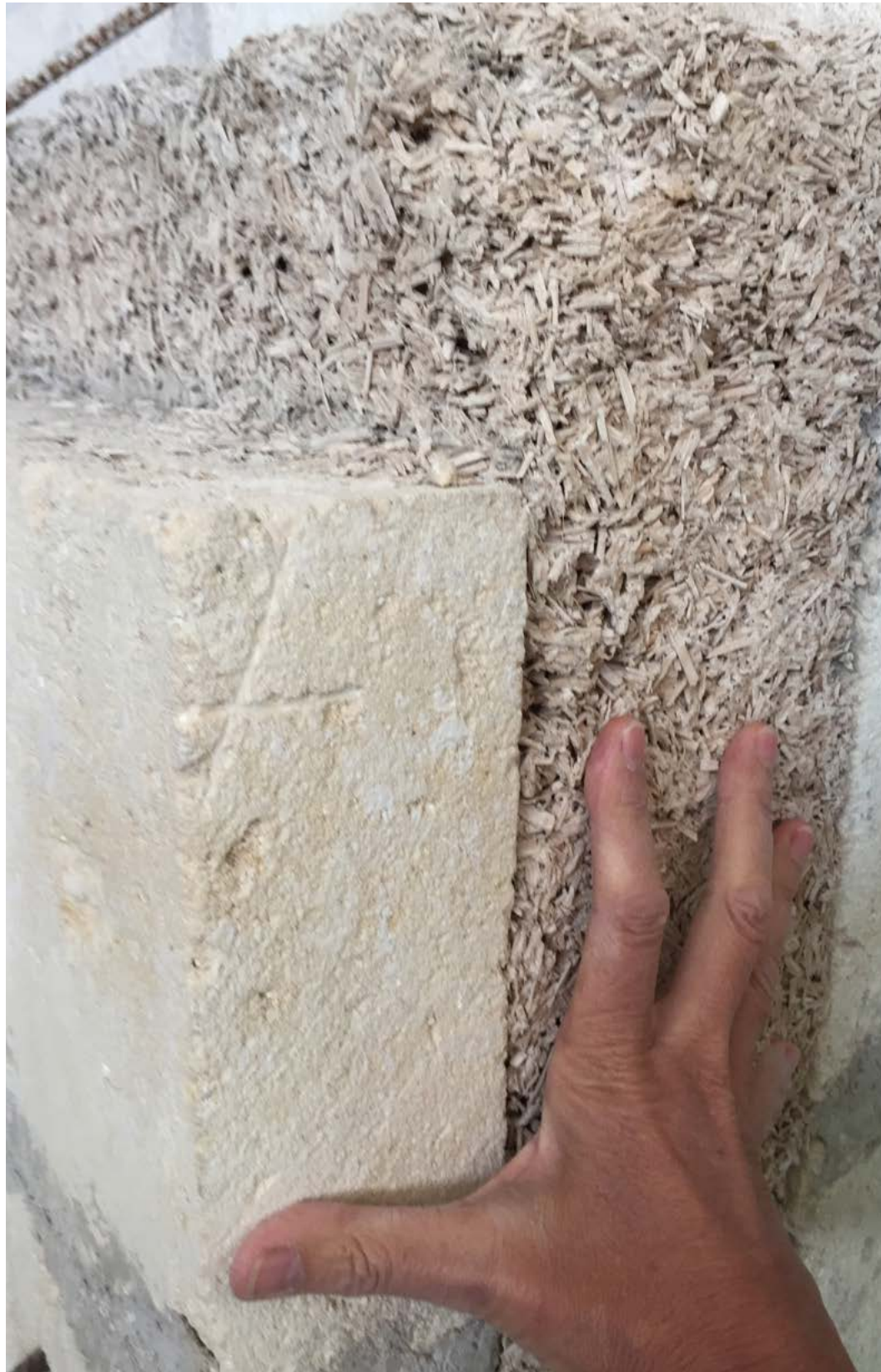
Fig 6.15 Masonry block and hemp and lime insulation
