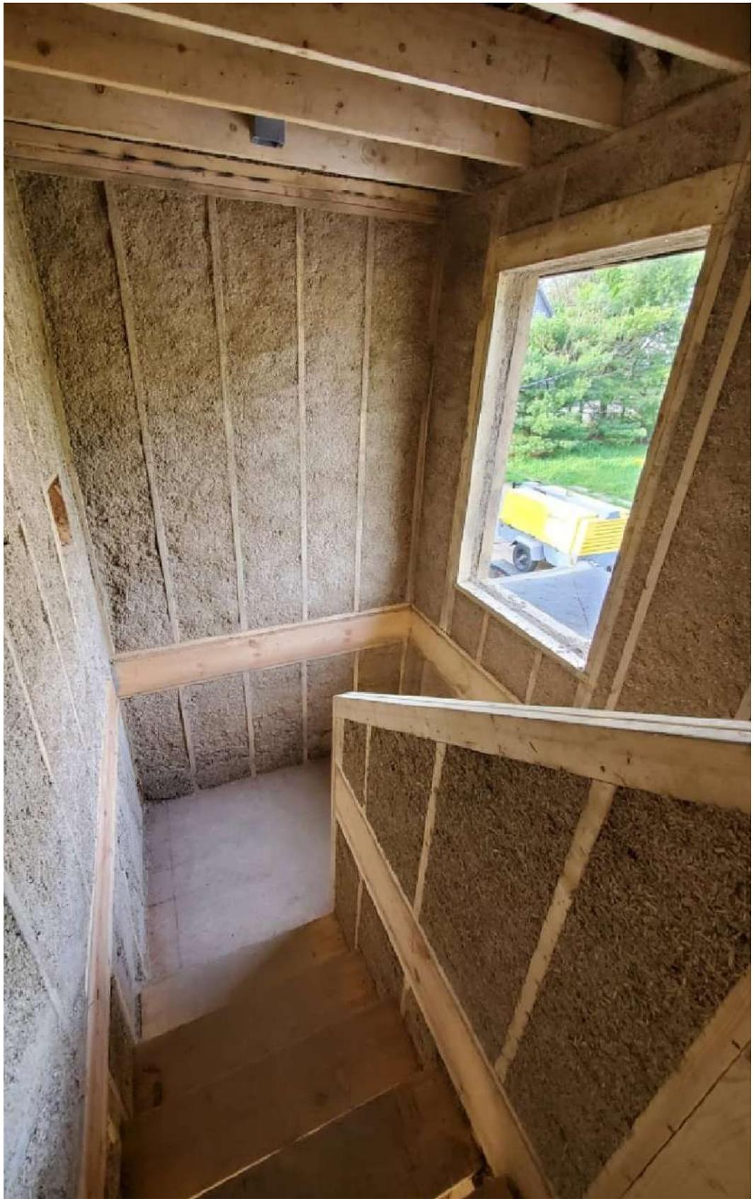
**Fig 5.16** The stairwell of PA Hemp Home with fully installed hemp
