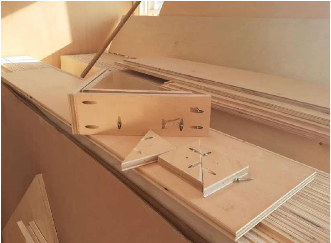
**Fig 6.3** Metal fasteners are being used rather than harmful adhesives
