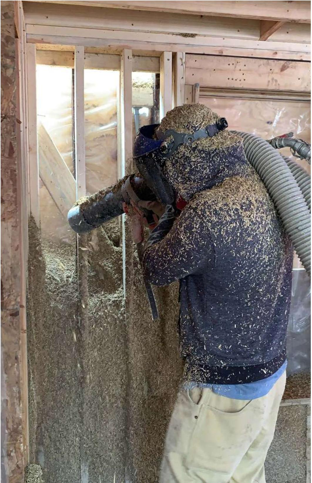
**Fig 5.11** Cameron from Americanvire installing the hemplime mixture
