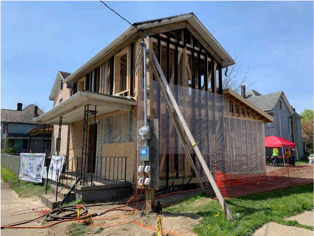
**Fig 5.6** The home fully framed and prepped for the spray-applied hemplime install
