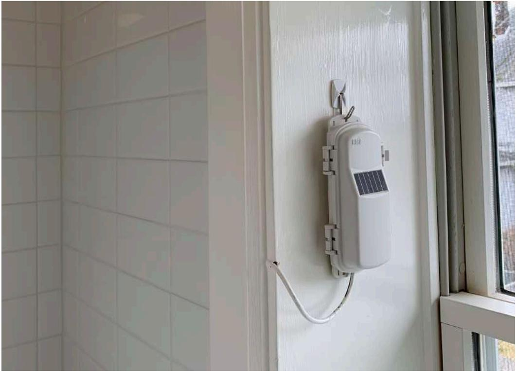
**Fig 8.4** Heat flux monitor in the upstairs bathroom that was installed by PHRC
