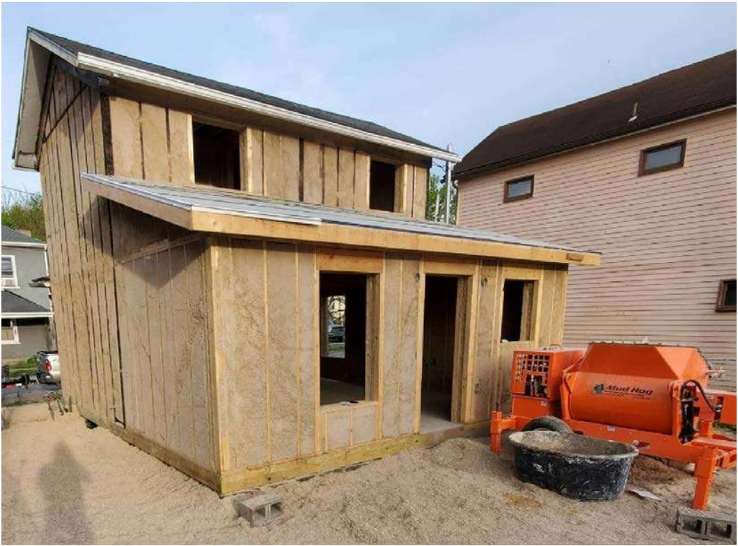
**Fig 5.15** PA Hemp Home after the hemp installation was completed
