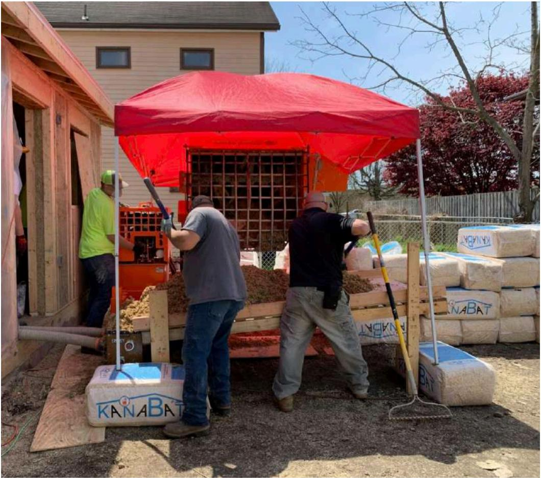
**Fig 5.12** The mixture comes out of the Mud-Hod onto a platform, where the team takes shovels to feed it into the sprayer
