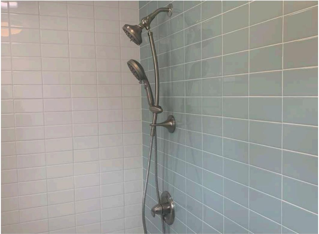
**Fig 6.8** Daltile Colorbody Porcelain in Waterfall used in the downstairs half-bathroom
