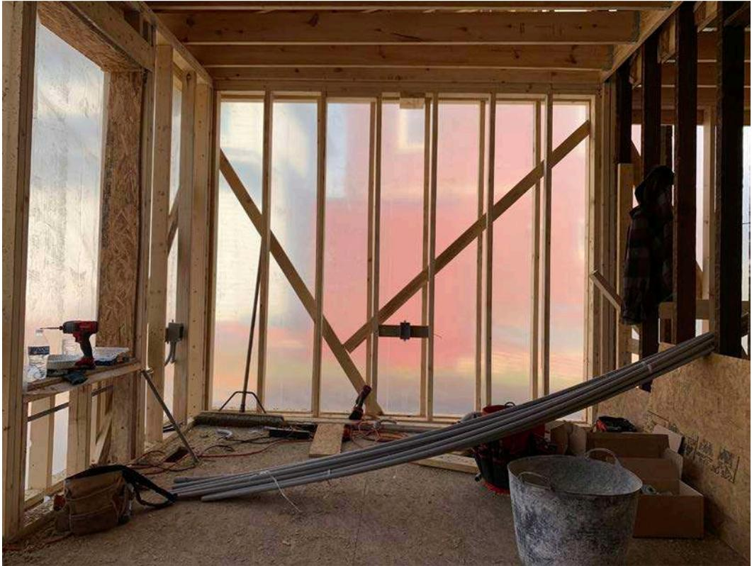
**Fig 5.2** (Left) Framing of the interior and exterior walls upstairs
