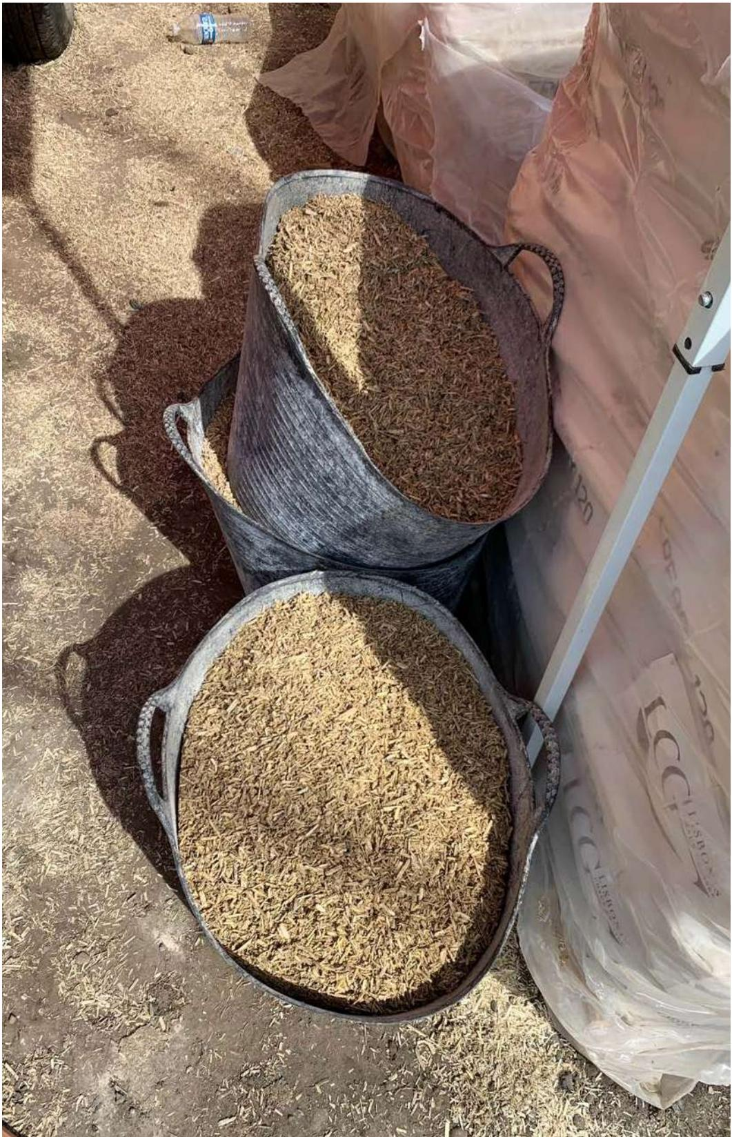
**Fig 5.14** The excess mixture can be re-added to the Mud Hog, leaving no waste behind
