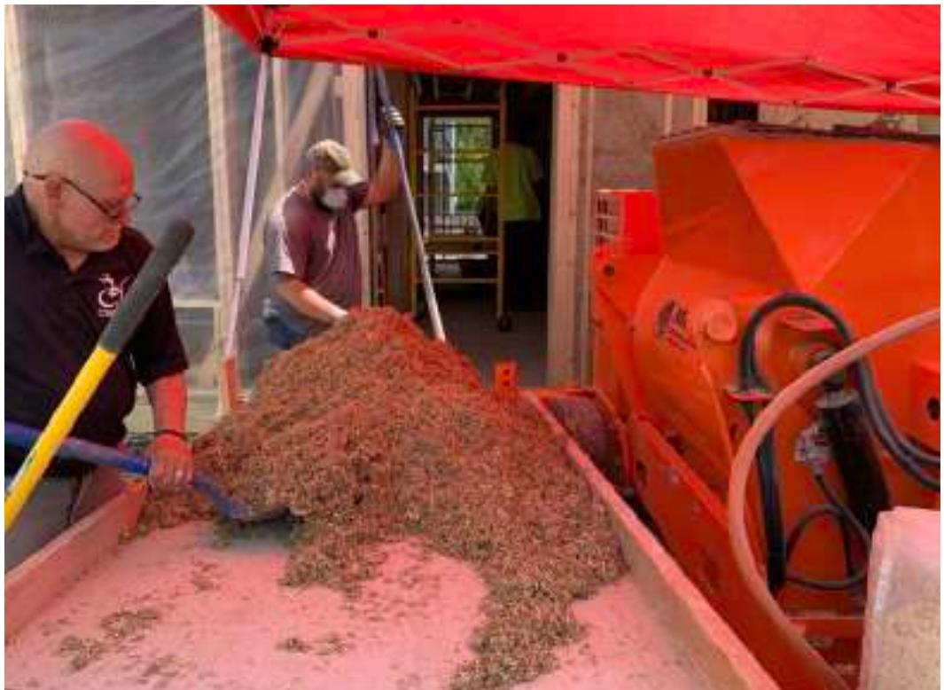
**Fig 5.9** The team then shovels the mixture from the Mud Hog, into the sprayer
