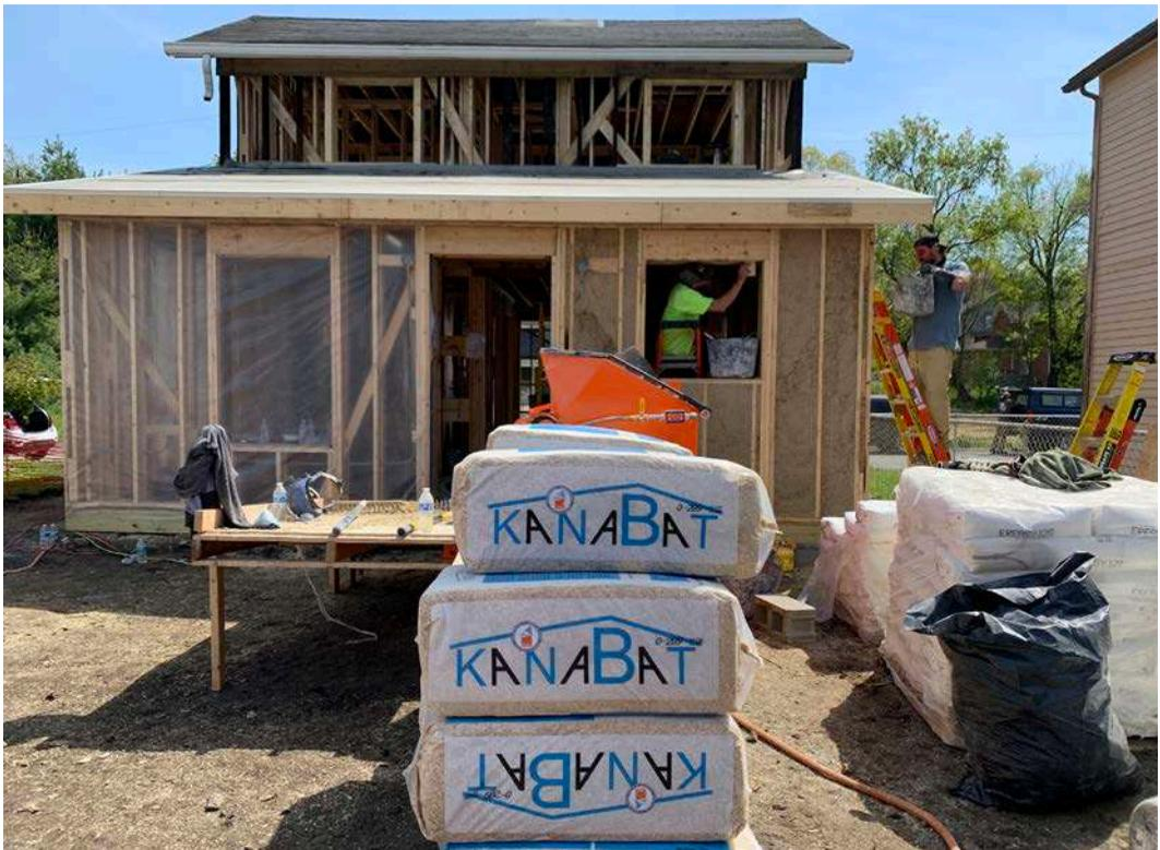
Fig 5.5 KanaBat is building grade Hemp hurd that will be mixed with Lime and Water
