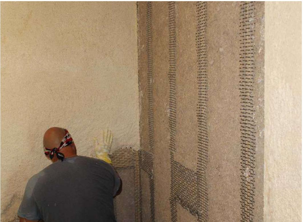
**Fig 5.21** Plaster mixture being installed in the downstairs bathroom
