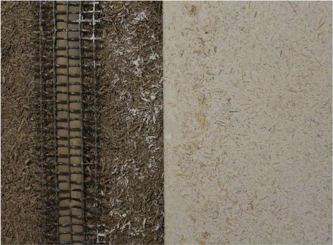
**Fig 5.22** Close up of hemplime, Exposed wood studs covered with lath and Plaster
