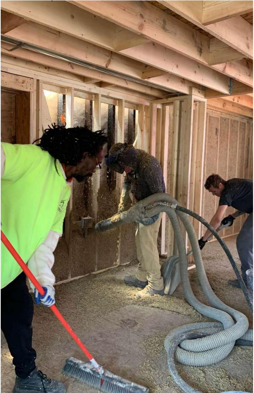
**Fig 5.13** On the inside, as the mixture is being installed, a team of two sweeps up the excess and shovels it into a buckets
