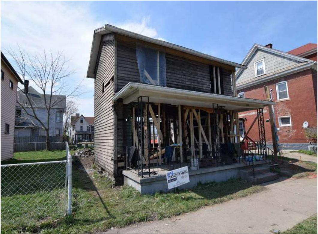
**Fig 4.6** Front of PA Hemp Home with the exterior siding stripped off and windows removed
