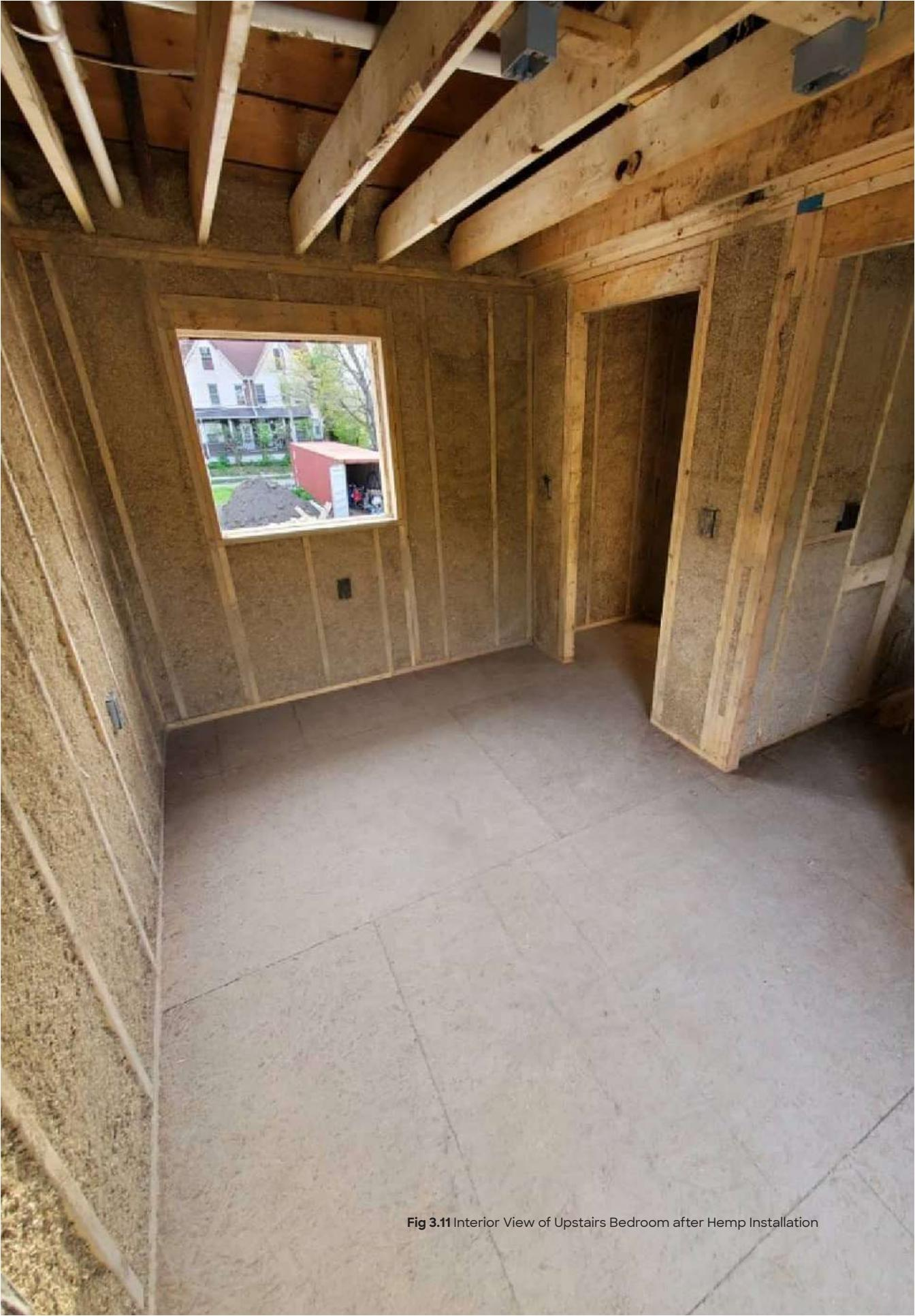
Fig 3.11 Interior View of Upstairs Bedroom after Hemp Installation
