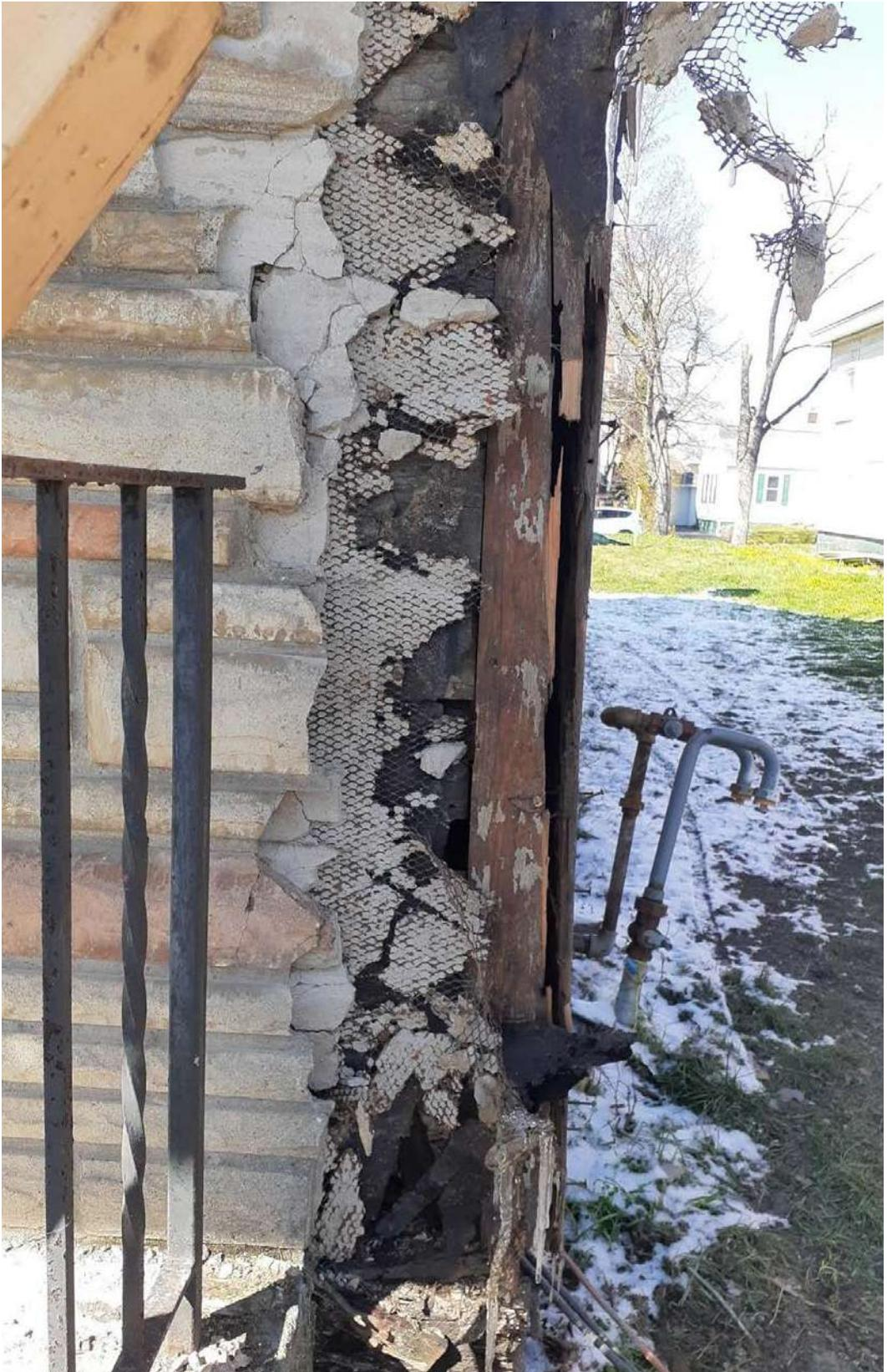
**Fig 4.9** Damaged wood and structure at the foundation
