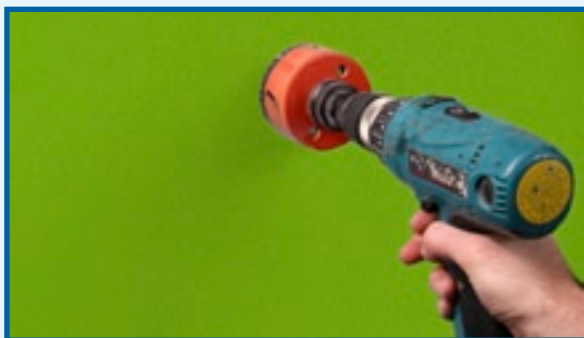
3. Drill a hole for the plug socket, install the wall socket.
