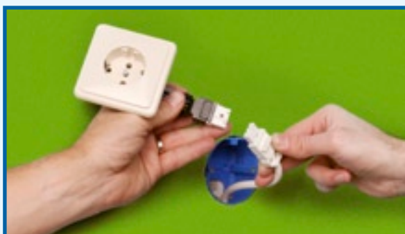
5. Install the plug socket and connect the wiring.
