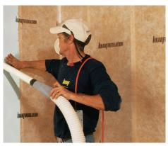
Jet Stream **ULTRA** is an excellent product for Blow-in-Blanket applications. It will dense-pack in wall cavities with no settling.
