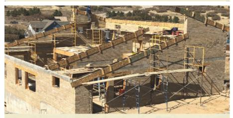
Exterior walls under construction with formwork for poured, reinforced concrete bond beam at the top of the wall and between floor levels.
