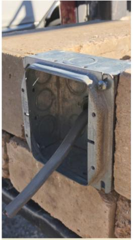
Electrical box placed in the wall during construction with conduit placed between the two whythes of blocks.
